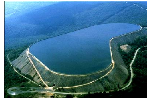
Pumped Hydro (Taum Sauk) 400 MW
