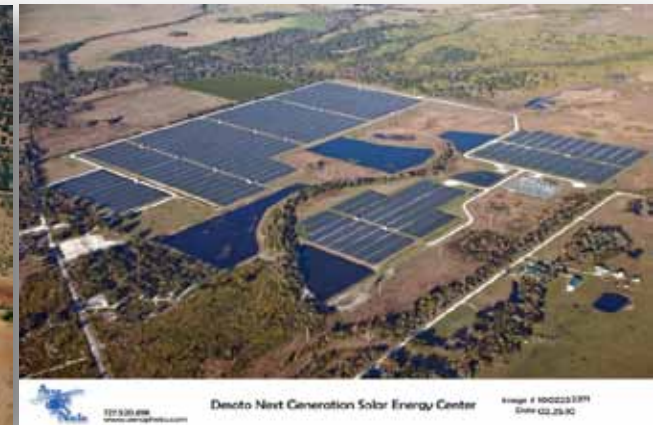
FPL Desoto, Florida, 25 MW SunPower T0 Tracker © 2010 SunPower Corporation
