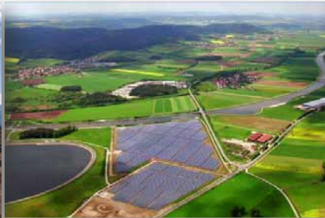
Bavaria Solar I&II, Germany, 10 MW SunPower T0 Tracker
