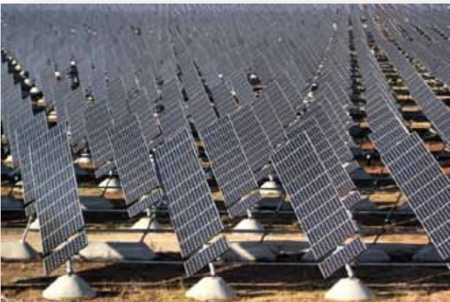
Olivenza, Spain 18 MW SunPower T0/T20 Tracker
