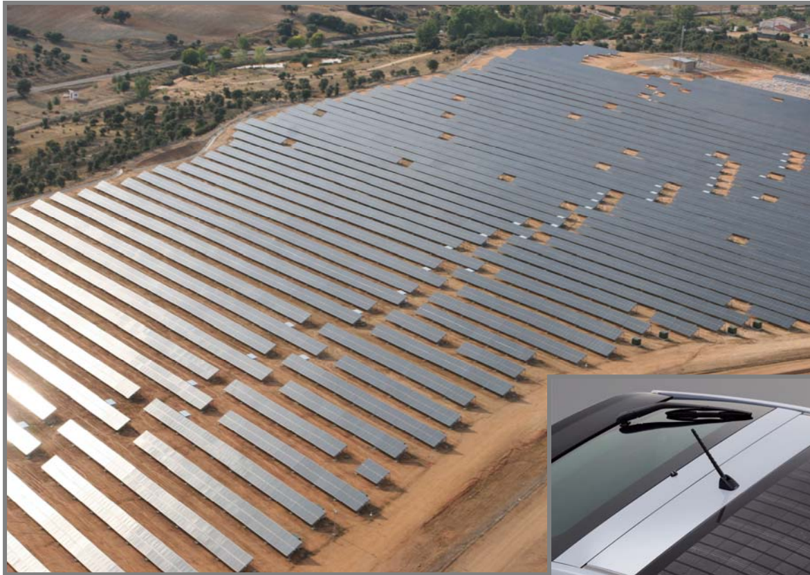
Avanzalia Solar, Spain
